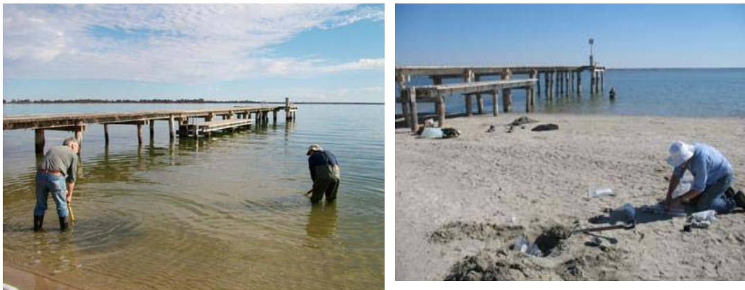
Figure 6. Changes in water level at Lake Bonney caused by isolating it from the Murray River using a temporary embankment to generate water savings in order to help mitigate drought-related problems in the MDB. Clockwise from above: July 2007 (showing mobilising of black monosulfides with water disturbance) to drying in April 2008, which shows white salt efflorescences comprising thenardite ( \text{Na}_2\text{SO}_4 ) and minor amounts of eugsterite (Na-Ca-sulfate mineral) along the beach at Barmera (Site F5 in Fig. 5). (from Fitzpatrick et al. 2008g)
