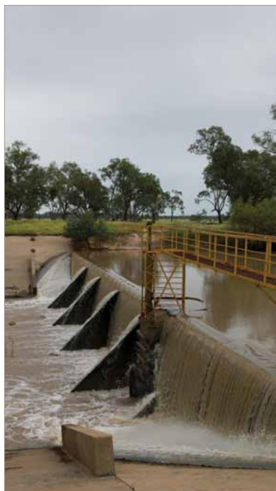
Weir on the Culgoa River, Queensland
