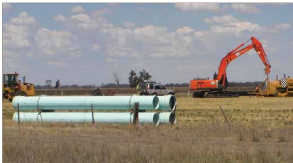
Wimmera Mallee Pipeline construction, Victoria
